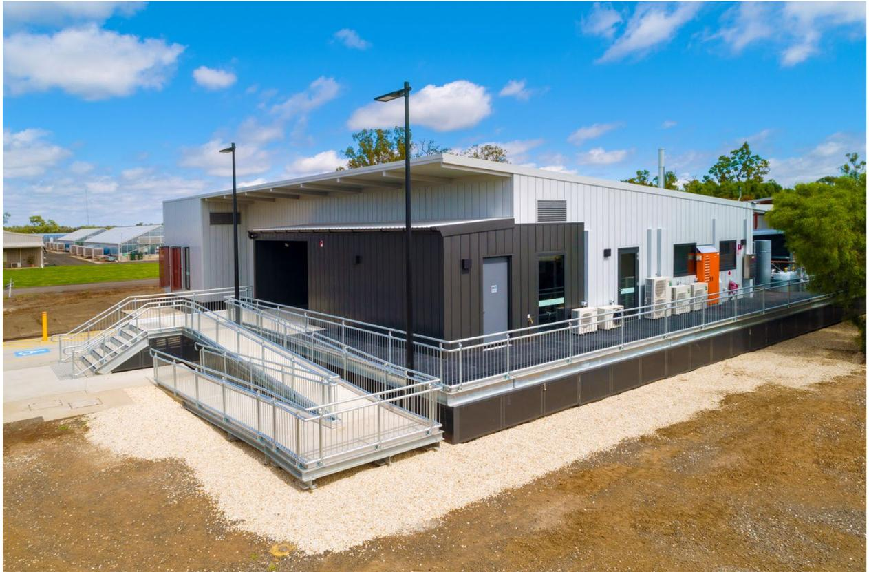
The laboratory was constructed using a non-traditional modular building solution. This solution involved off-site fabrication, with the remaining works undertaken onsite in a similar fashion to traditional construction methodology—all within an operational environment.
