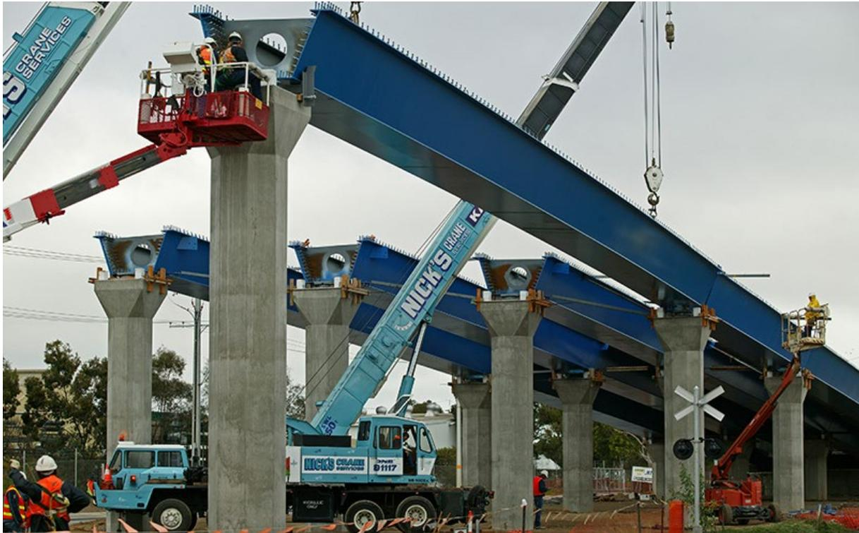
Planning for erection should start at the very beginning of the design process. Such planning should consider the construction sequence, the design factors that affect buildability and site practice in terms of typical erection plant.
