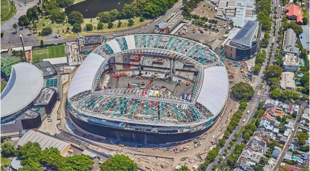
The 'Pringle' shaped roof sits atop the coliseum like 'bowl' steel structure, which simultaneously supports the pre-cast tiered seating for 42,500 enthusiastic cheering fans.
