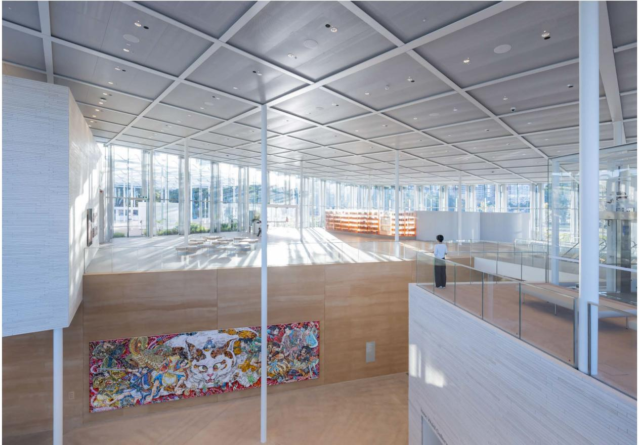
The design transforms the southern of the two fuel tanks into a unique art space of 2,200m<sup>2</sup>. The intent of the art gallery was for this space to be left 'raw', with the only spatial interventions being a new floor and drainage, new openings cut into the walls for egress, and a spiral stair inserted through a circular penetration in the roof.
