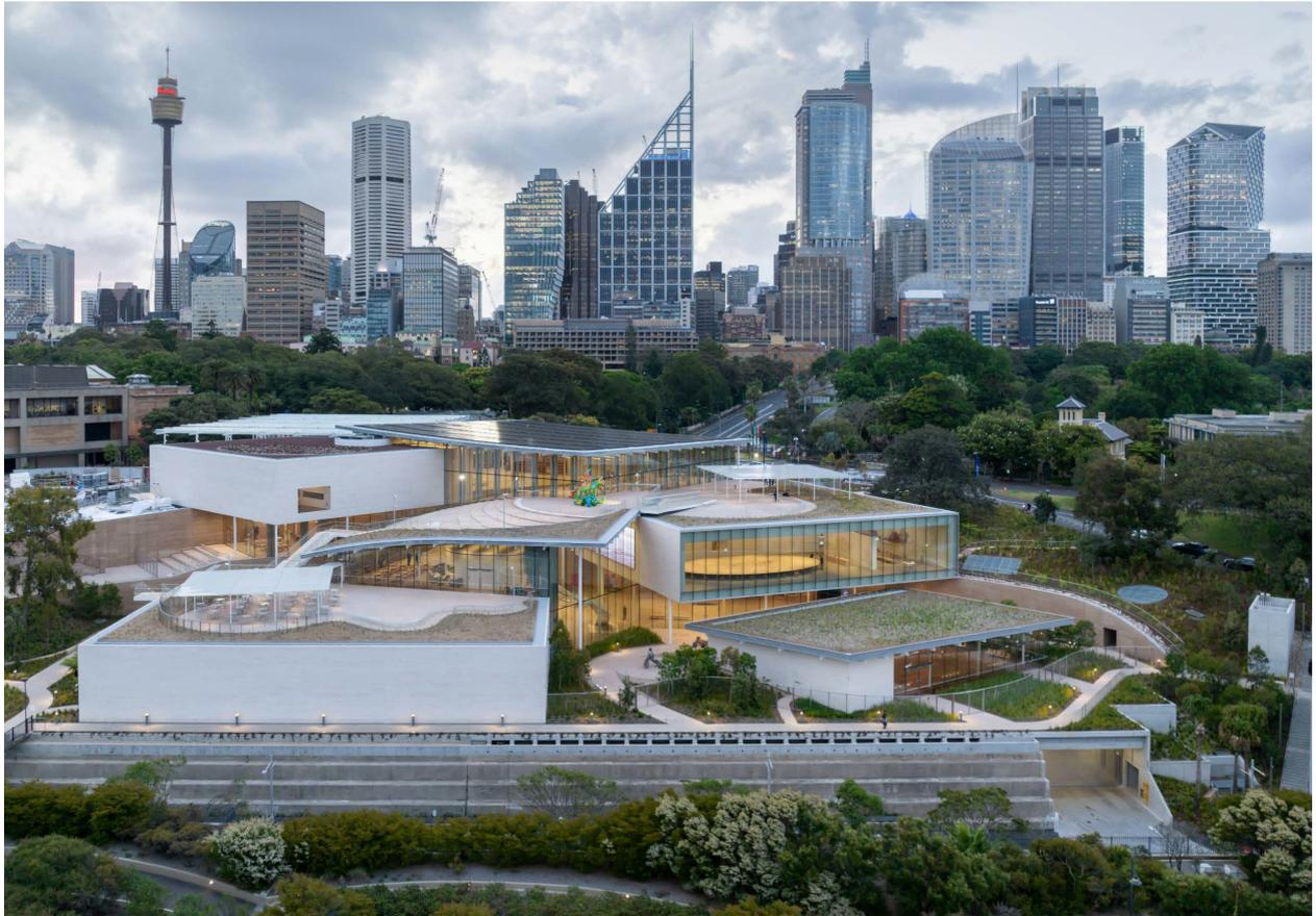
Adding complexity was a pair of decommissioned Navy fuel tanks below the site, built during WWII in a former sandstone quarry. The new building is formed from interlocking art pavilions nestled into the landscape over five levels, resting lightly on the land bridge and the fuel tanks. Each pavilion connects with the outdoors, via roof terraces, walkways, and landscaped gardens.
