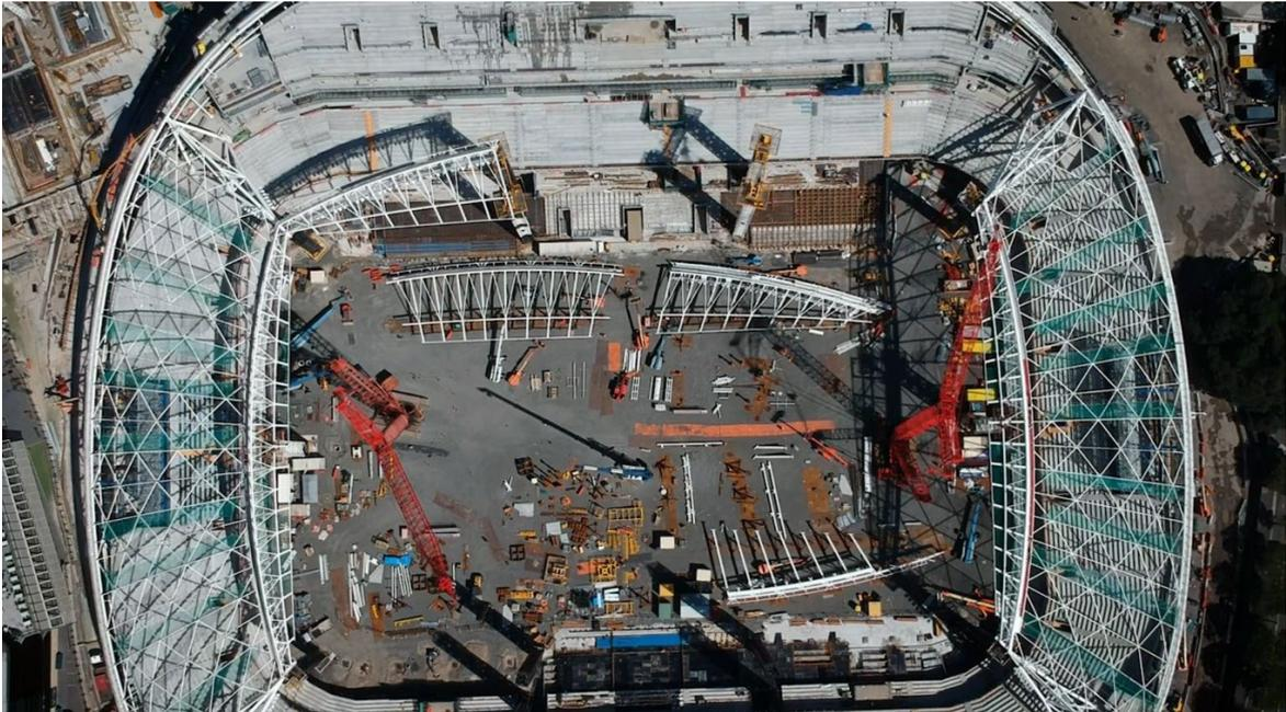
S&L Steel, both SCA and ESC certified, was awarded the contract to fabricate the complex roof structure, which consisted of a tension ring located on the outside perimeter of the roof, four derricks which support the roof in the four corners and four trusses broken into ten liftable sections which are complemented by the diagrid structure being a combination of RHS, CHS and plated node connections.
