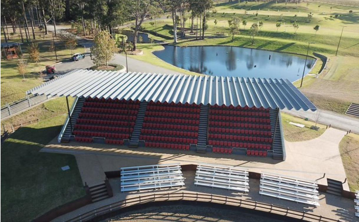
ARAMAX wide span roofing is rolled on site. Image courtesy Bay & Coast Metal Roofing.
