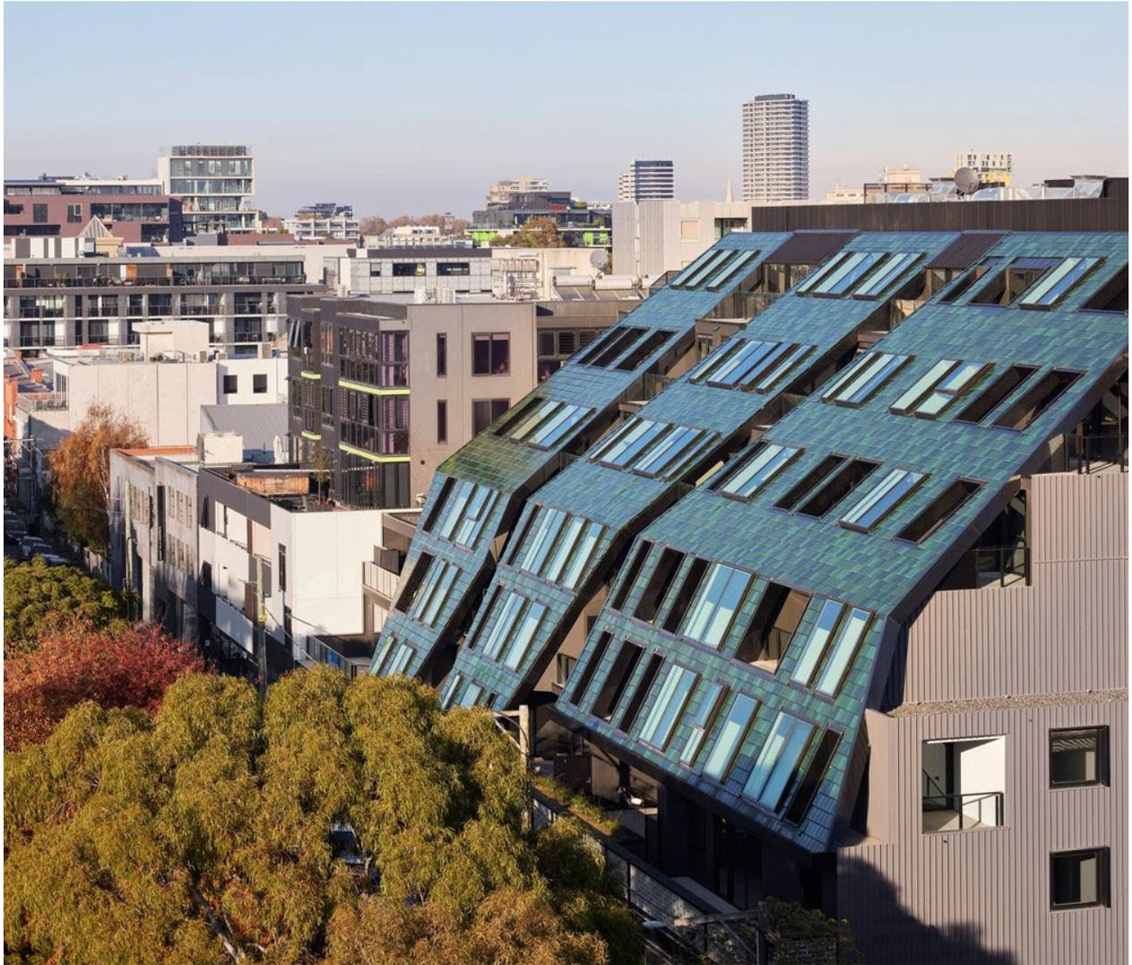
The project's custom-built blue steel truss system, developed by Bolt Blue Constructions and Dynamic Steel Frame, ensured adequate stability for both the thousands of tiles and large windows – some weighing over 500kg – while allowing for immersive views of the skyline. The truss system is fixed to posttensioned slabs, which allowed greater flexibility in achieving the unique design whilst also ensuring rigidity.
