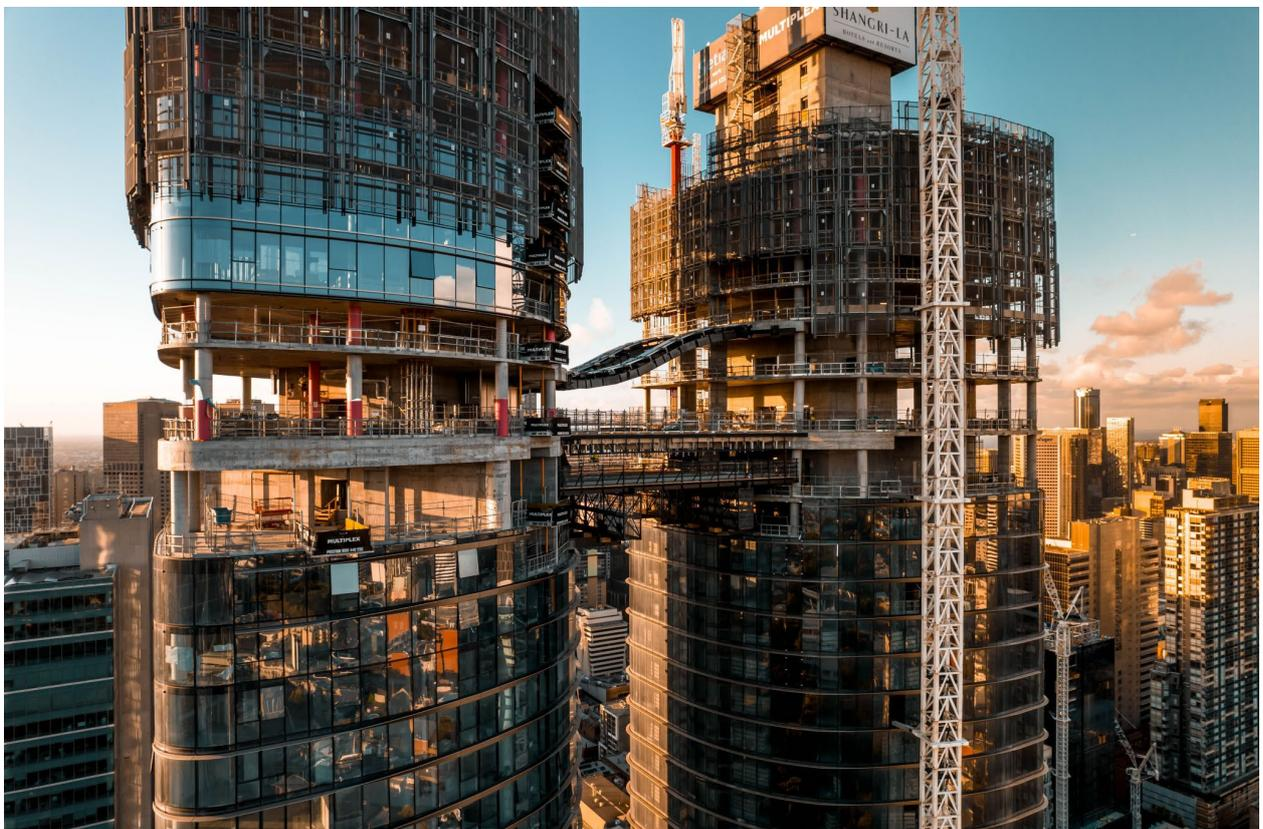
The main works for the project commenced with one of the largest concrete pours in Melbourne's history—a day long concrete raft pour covering an area of 1,000m<sup>2</sup>. This monumental 3m deep raft foundation is located on top of an existing railway tunnel and supports the new landmark mixed-use precinct.
