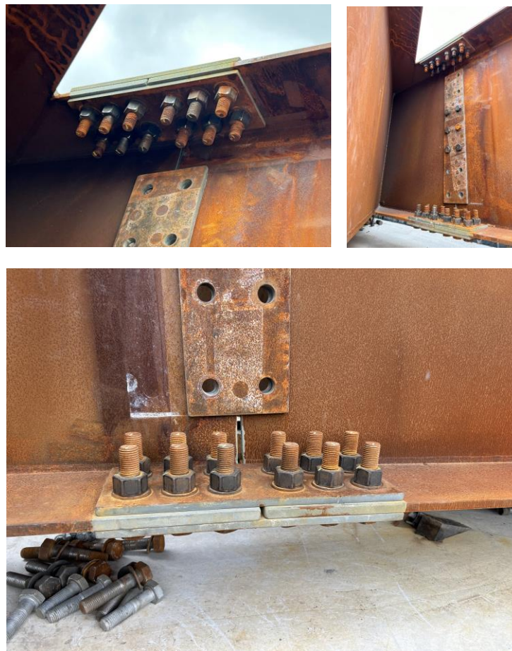
Figure 31 Weathering steel bolts unable to be tensioned due to poor site handling practice
