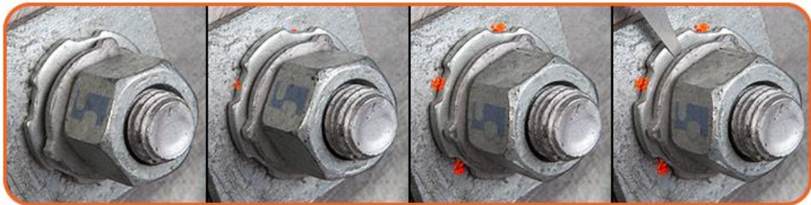
Figure 24 Example compressible washer type DTI's
