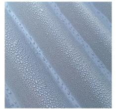
Exposure to clear night skies can cause the surface temperature of the metal roof to fall below the dew point, and moisture contained in the external air will condense on the roof surface.
