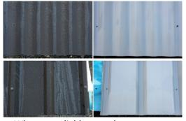
Where a pliable membrane vapour barrier is installed underneath metal roofing and draped to create an air gap to thermally protect from the cold roof sheet, the possibility of internal moisture reaching the underside of the metal roof sheeting is further restricted.
