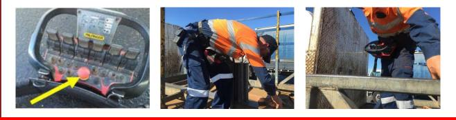
On the 30/10/2015 a worker delivering steel reinforcing products was struck by a vehicle mounted crane, the worker was using a remote control at the time of the incident and was on the vehicle tray balancing the load/lifting equipment prior to making the final lift.
