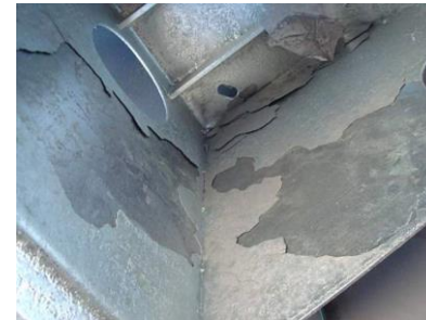
Poor galvanising results
