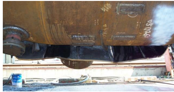
Pressure vessel cracking
